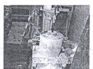
Figure 3: Vibrating the concrete
